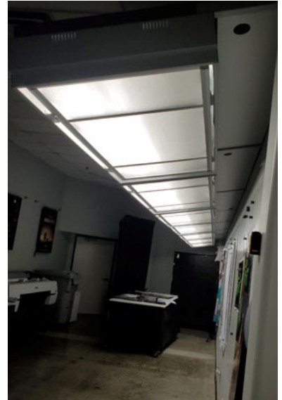
Midnight Oil has banks of five to seven luminaires placed throughout their facility.
