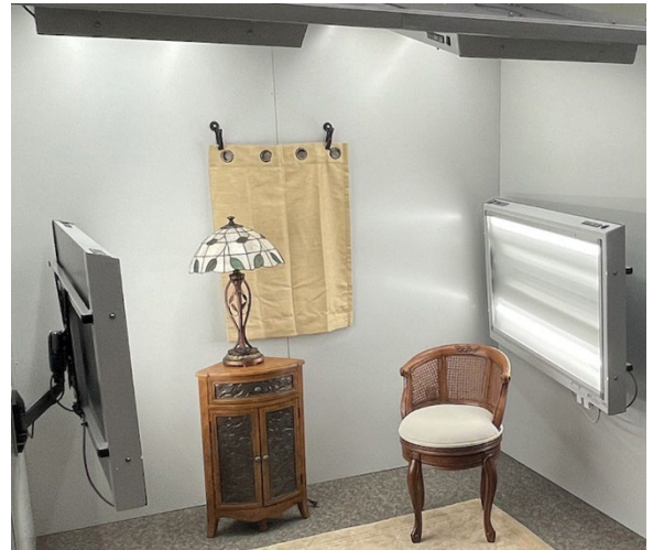
The combination of adjustable side luminaires and ceiling mounted luminaires allows Touch of Class to properly view a range of products at once.
